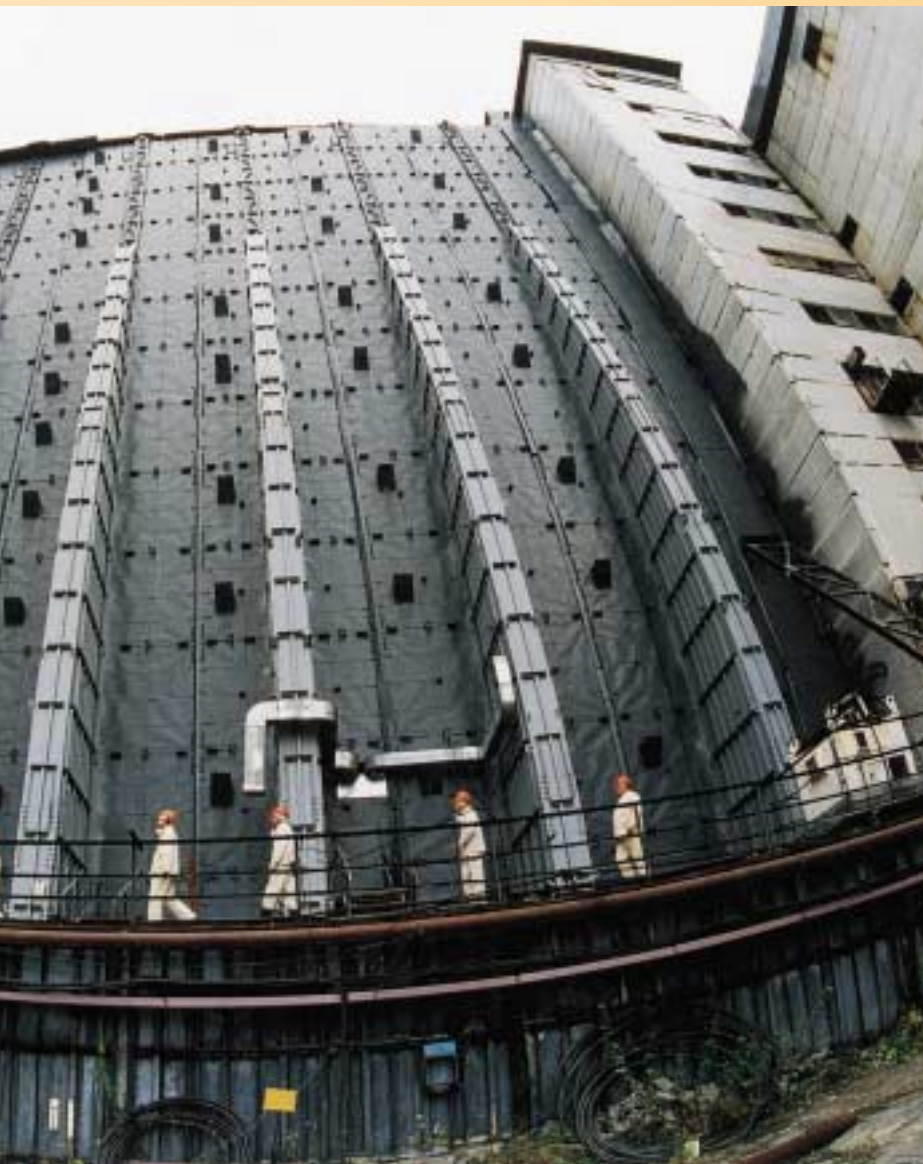
The butress wall of the shelter.
